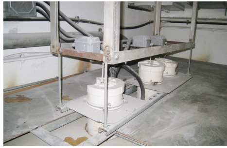
鞮鞮式水銀制 Swing type mercury switches
