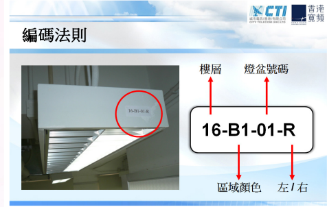
為加快確認維修保養項目，於物料標貼上的編碼法則。 The coding method on labels of materials for identifying repair and maintenance cases more easily.
