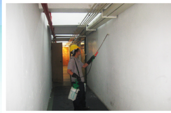
使用掃油器翻新牆身 Using "Paint Spraying Container" for painting wall
